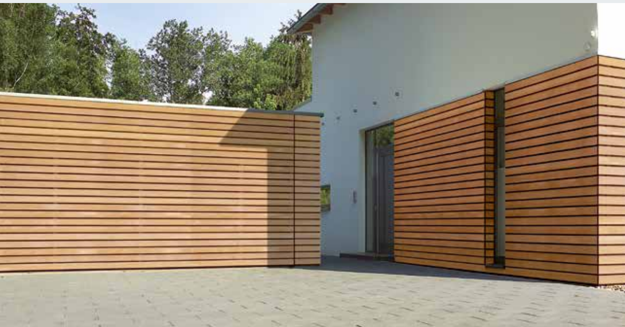
On-site cladding with timber panels
