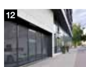
Collective garage doors
