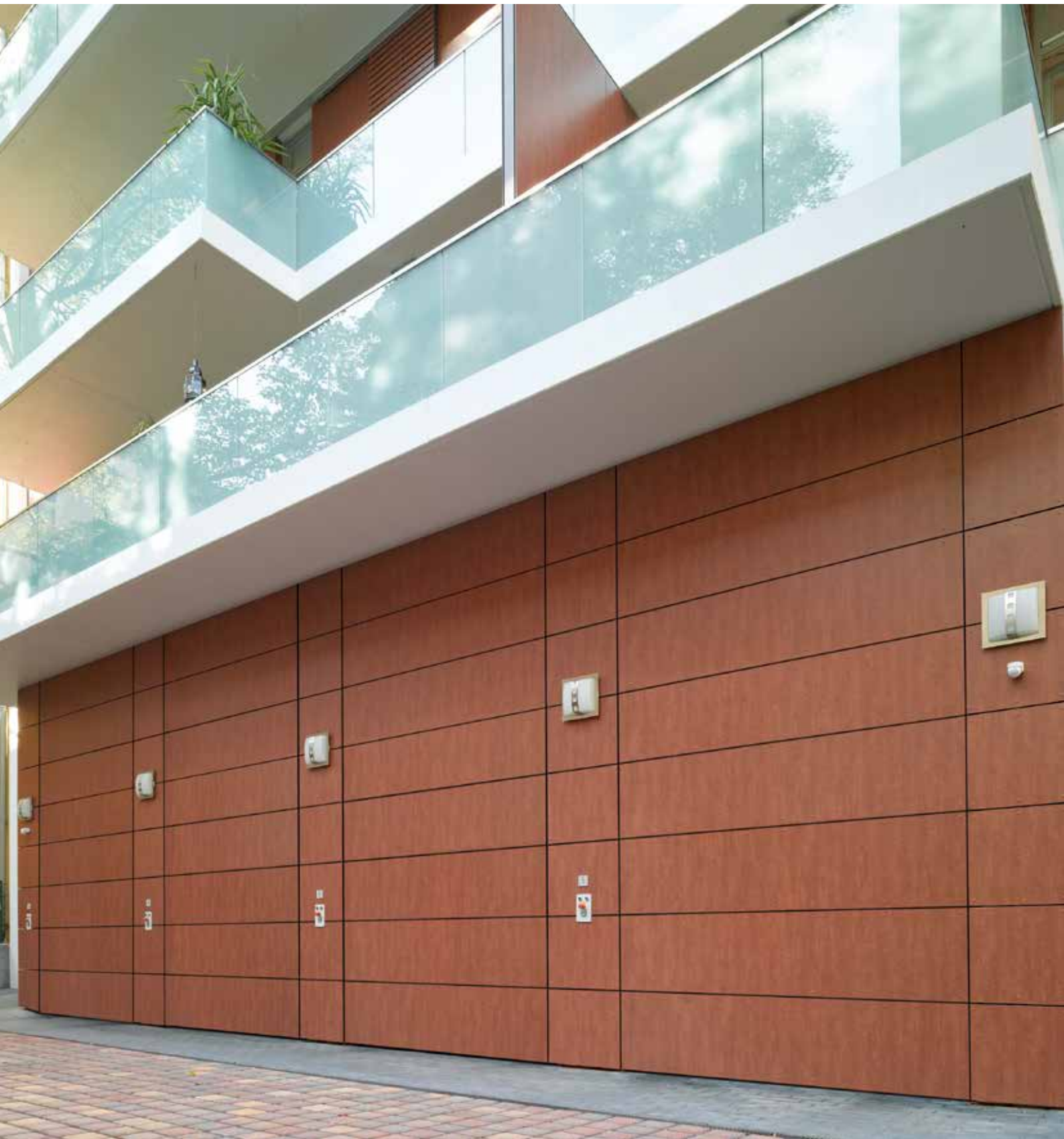
On-site cladding with laminated timber boards
