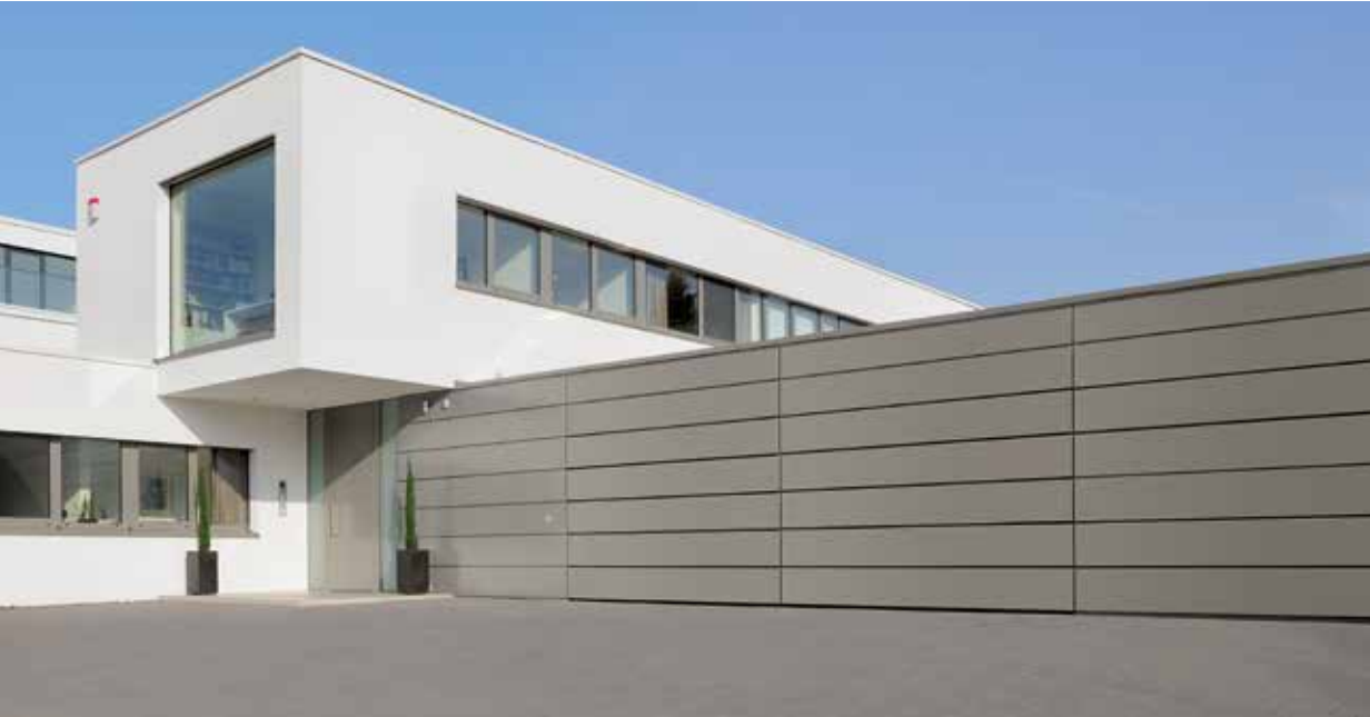
On-site cladding with aluminium compound board
